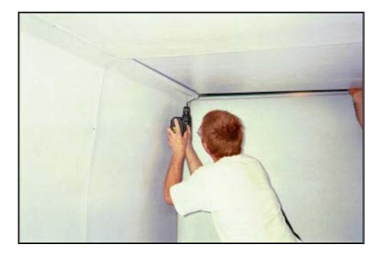
Secure bulkhead to driver side wall panel, roof, floor, and side door panels with #10 x 2.5" pan head screws. All holes to be drilled 5/32 inch.
