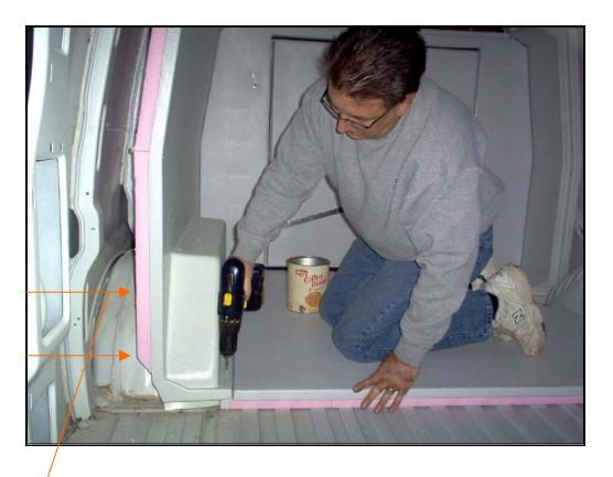
INSTALL TIP - BACK OF PANEL SHOULD BE PUSHED BY SECOND INSTALLER WHEN FIRST INSTALLER IS DRILLING HOLES FOR SCREWS TO ENSURE TIGHT JOINTS. Load rear roof panel part #VLS 002 through side door opening, slide into position on top of wheel arch panels until it mates in line with the floor and 11.5" wall panels.
